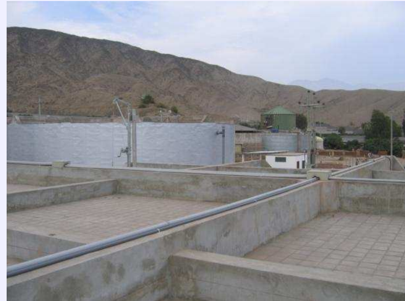
Digester with concrete roof and example of agitator
